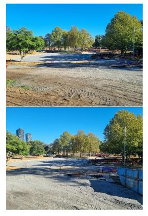
The Rymill Park lake base has been completed, the raingarden structures are constructed, and the underground storage tanks are progressing well.
